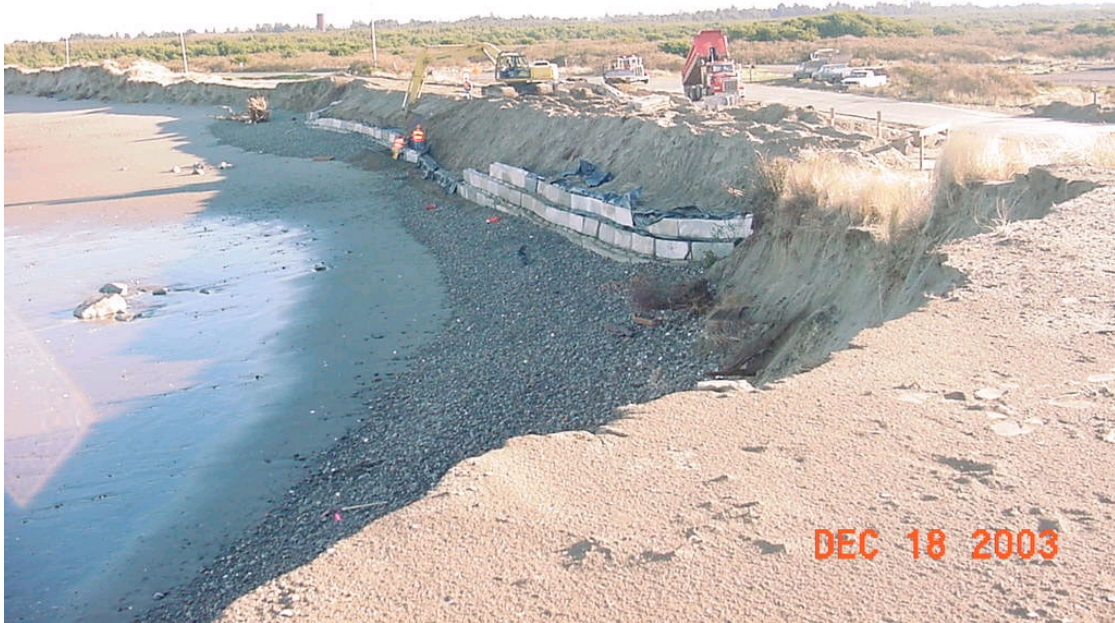
Figure 9: Photos of Westport's emergency shoreline armoring just west of project site, looking east. Cars to right are in Westhaven State Park parking lot. Erosion in front of condominium site is shown just beyond seawall construction site.
