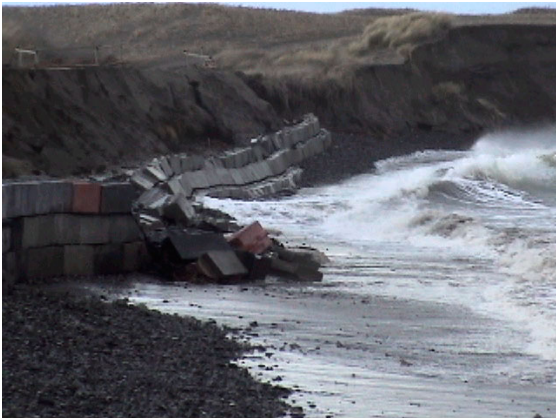
Figure 10. Erosion destroys the new seawall, looking west.
